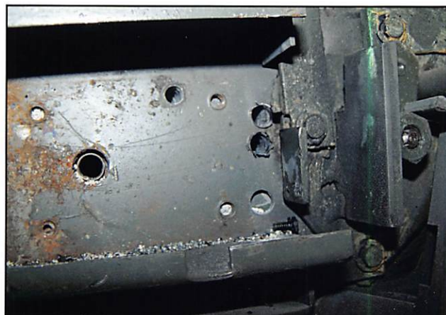
Photo 6 show the lock mounting surface with the 3 holes drilled, two at the bolt and the third for the relock.
